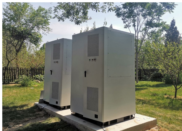
Electric vehicle charging station, 460kWh.
