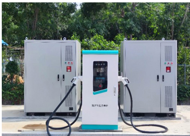
Switching station area, 50 sets of QC-215K-O.
