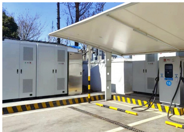
Electric vehicle charging station, 920kWh.
